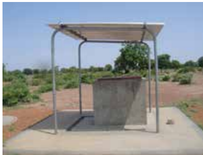
Construction de borne fontaine/AEP Diebougou Burkina Faso/2012-2013
