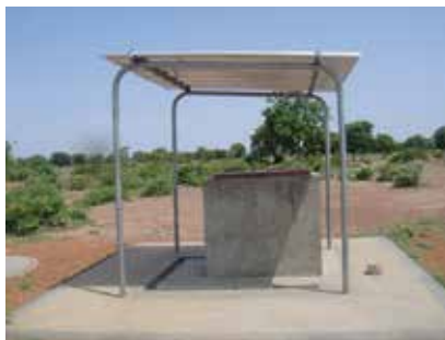
Construction de borne fontaine/AEP Diebougou Burkina Faso/2012-2013
