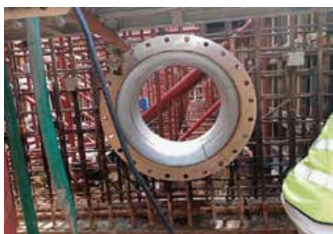
Pose de manchette inox reservoir 4500m 3 /PAEP Bamako-Kabala/ Mali/2018-2021
